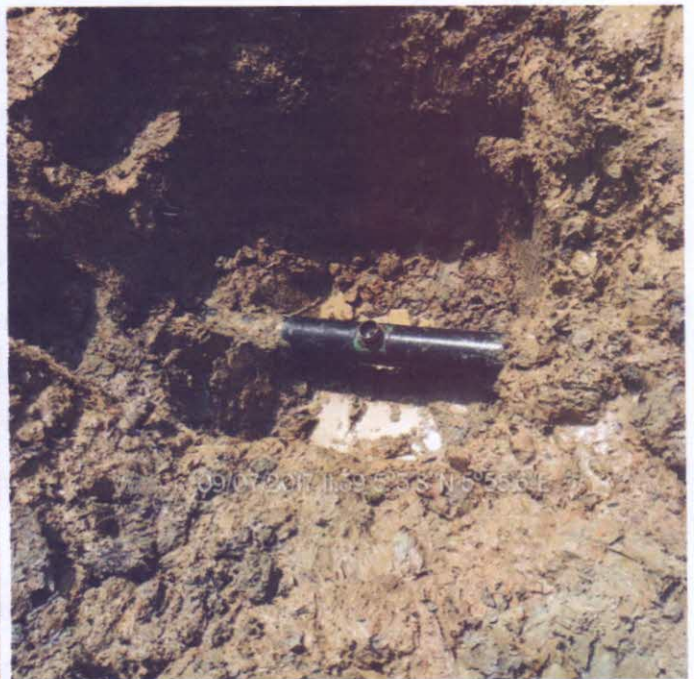
Fig B: Incident Facility after excavation
