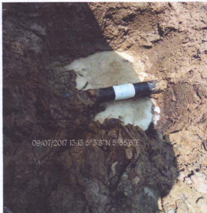
Fig C: Incident facility after repair
